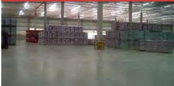
Sumaré Warehouse in Brazil
