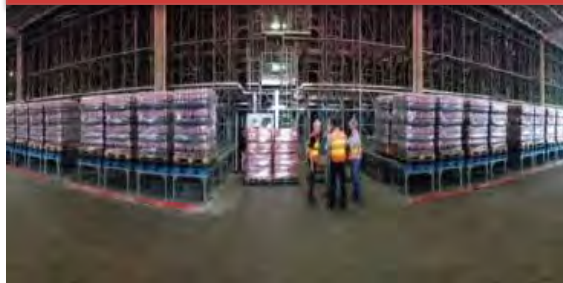
Jundai Vertical Warehouse in Brazil
